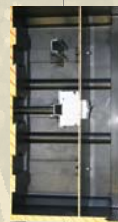
rail support system and cover panel for fuses
